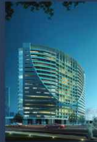
The V Tower
